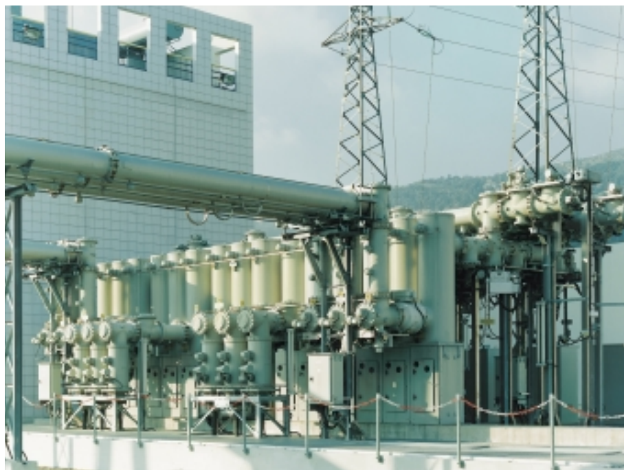
fig. 7 SF 6 switching station, 245 kV (Schneider Electric High Voltage, France)
