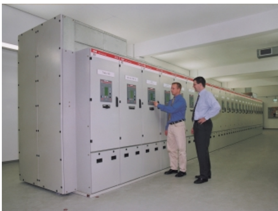
fig. 12 Metal-clad SF 6 -insulated switching station in a compact design (ABB Calor Emag, Germany)
