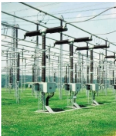
fig. 6 Outdoor transforming station with SF 6 equipment, 420 kV (Siemens, Germany)
