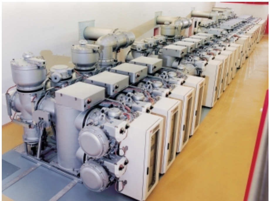
fig. 1 Enclosed, \text{SF}_6 -insulated, high-voltage plant (ABB, Switzerland)
