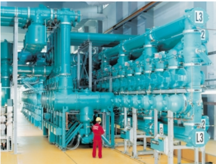
fig. 5 Gas insulated High-voltage switching station, 550 kV (Siemens, Germany)
