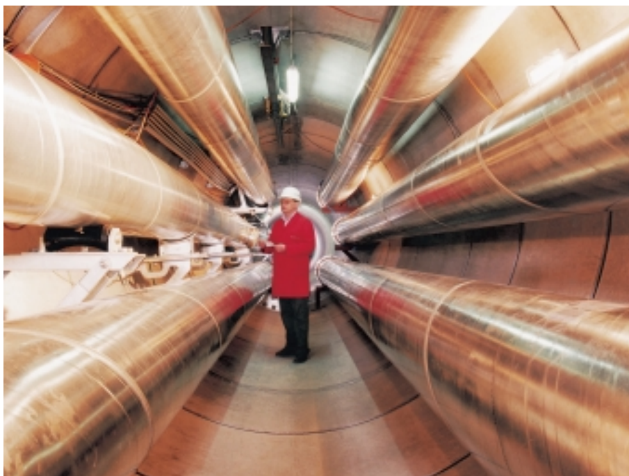
fig. 10 \text{SF}_6/\text{N}_2 mixture in transmission lines, in tunnel (Siemens, Germany)
