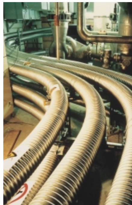
fig. 14 SF 6 -insulated high-voltage cable in the JET nuclear-fusion plant (kabelmetal electro, Germany)
