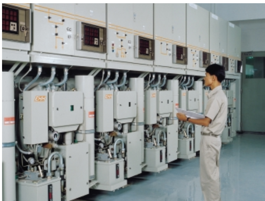
fig. 2 SF 6 -insulated high-voltage switching station type L-SEP, 145 kV (VA Tech Elin Holec High Voltage, Netherlands)
