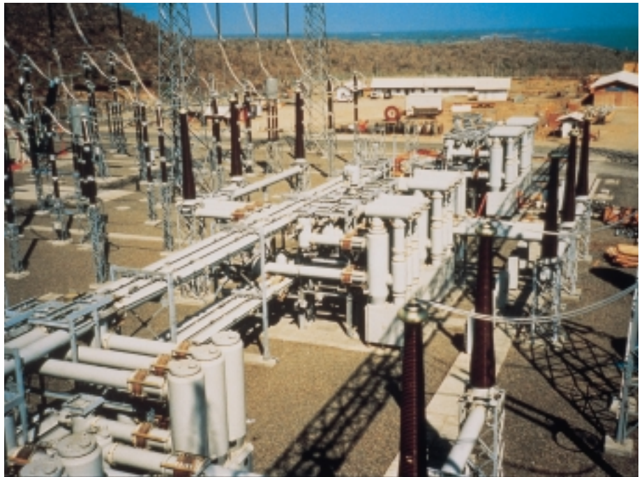
fig. 4 Enclosed switching station, 500 kV (Alstom, France)
